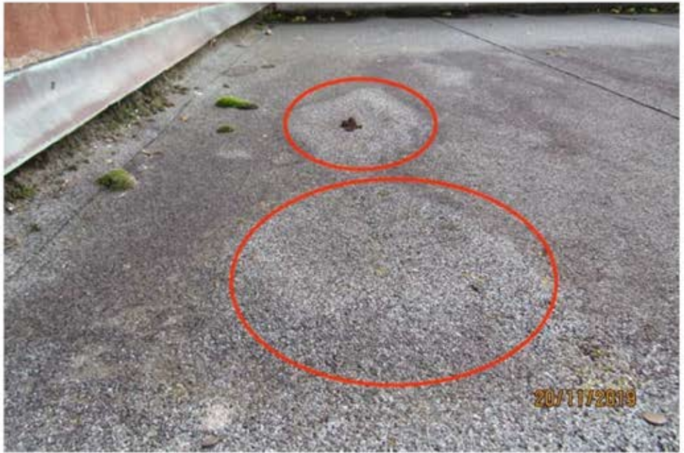
Raised areas of flat roof felt
