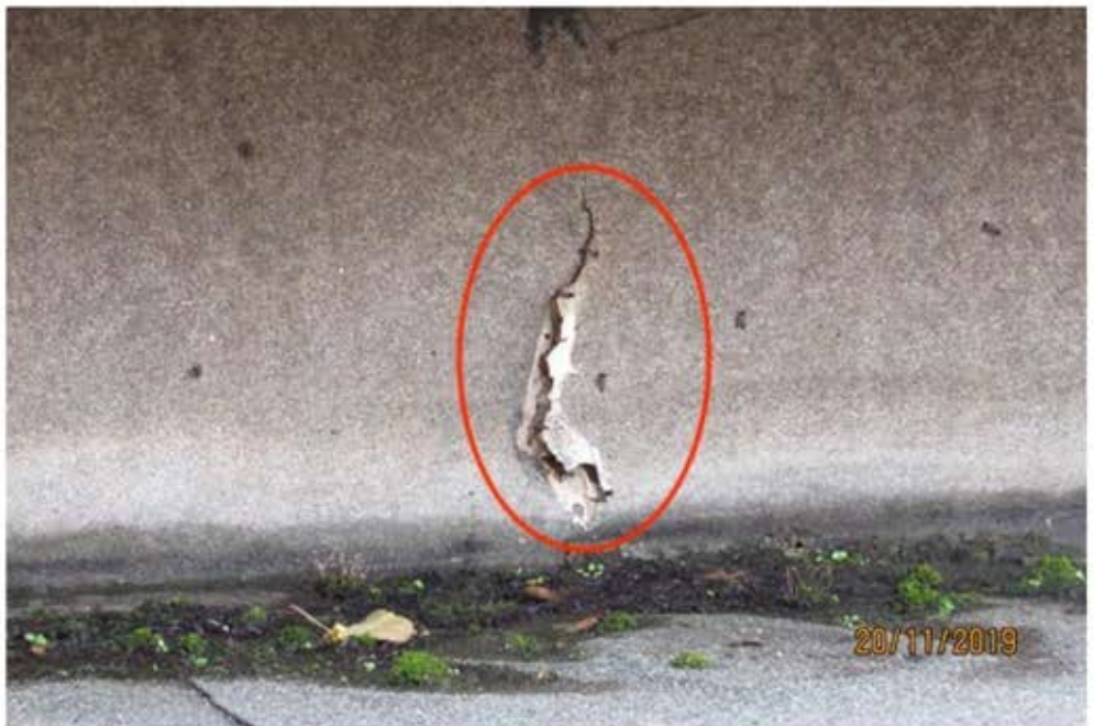
Damaged felt on wall between flat roof and lean-to roof
