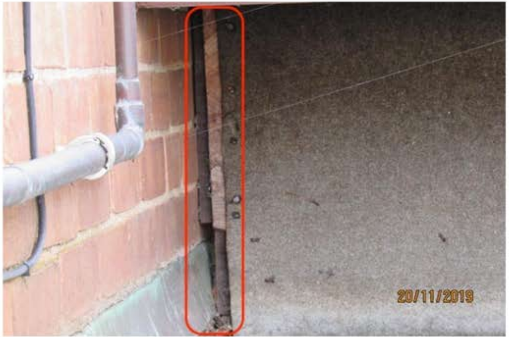
Insufficient abutment of roof felt on wall between flat roof and lean-to roof
