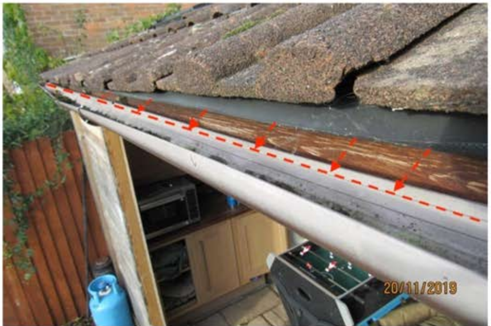
Incorrect position of lean-to roof underlay
