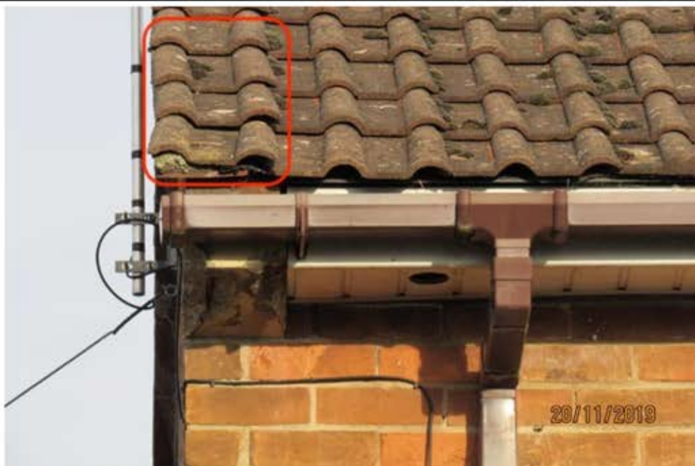
Misalignment of roof tiles above south-west corner
