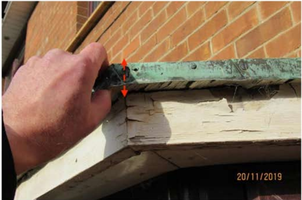
Bay window roof insufficiently fixed and timber frame decaying
