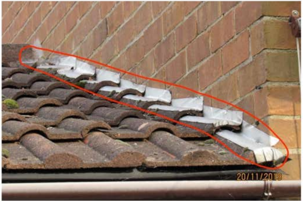
Flashband on lean-to roof
