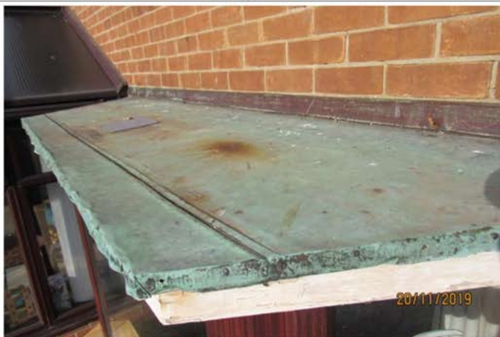
Weathered copper covering to bay window roof
