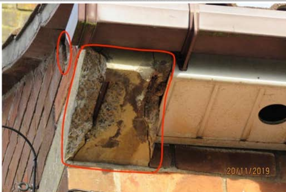
Severely damaged rear Corbel and opening between bricks above
